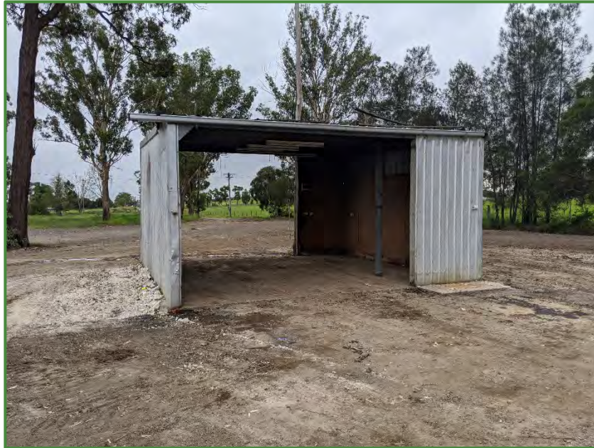
Photograph 7: Close up shed structure to be demolished. Looking north.
