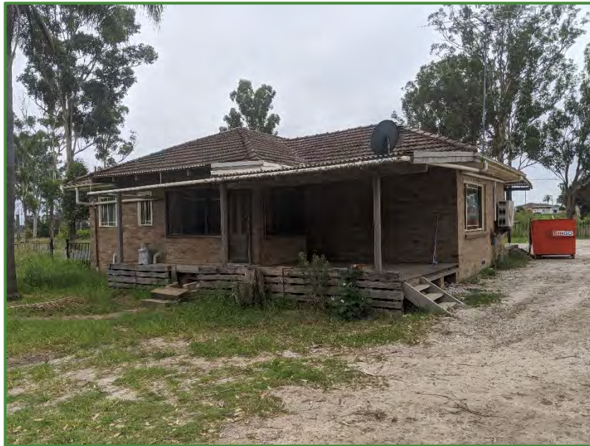
Photograph 5: Close up of residence structure to remain as on site office building. Looking east.
