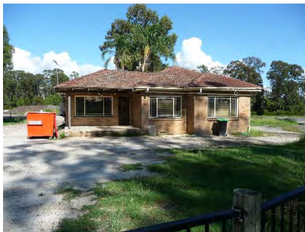
View to approximately southwest showing an existing building on the subject site to be converted into an office
