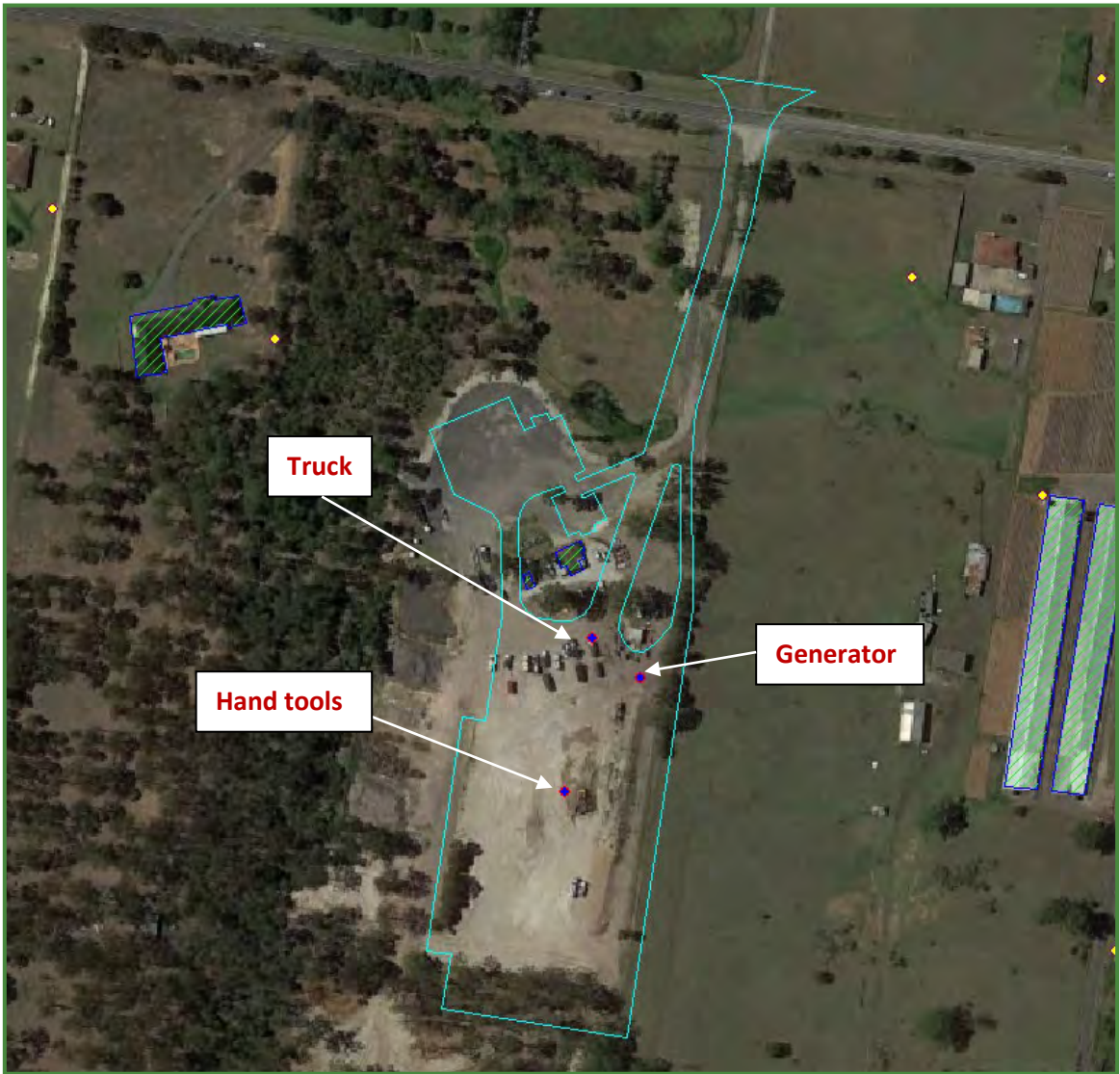
Figure 9-1: Construction Stage 1 – Site Establishment
