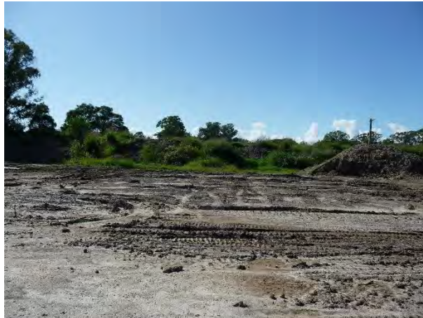
View to approximately east from the existing cleared area on the subject site showing the approximate position of the proposed waste recycling building
