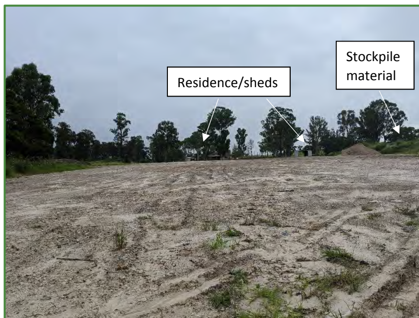
Photograph 18: Cleared extent of site. Note residence/sheds in centre and built up stockpile material on right of photograph. Looking north.
