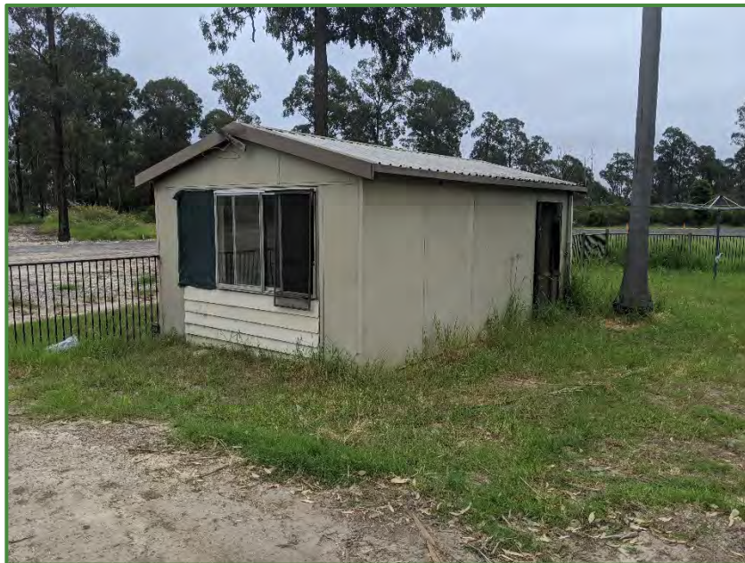
Photograph 6: Close up of shed structure associated with residence. Looking north.
