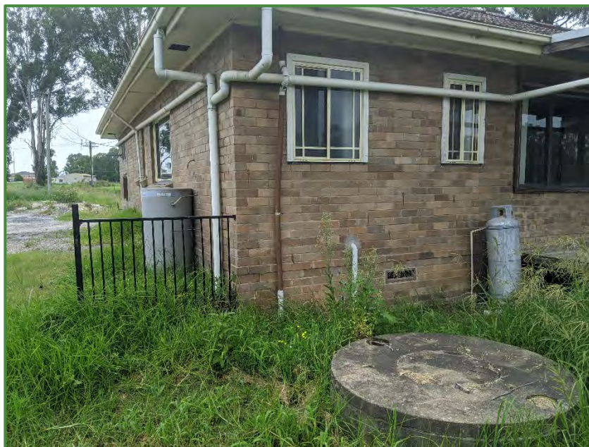
Photograph 8: Close up of septic tank associated with residence. Note water heating system and LPG cylinder attached to residence. Looking east.
